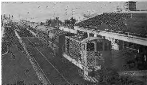
Above: Self portrait of Ben Byrne with retired locomotive No. 800 "Meadbe," Class B.L.A. 4-6-0, built in Ireland in 1939. Below: Diesel locomotive No. B-129, 960 h.p., built by General Motors in 1960. Passenger train is at Malabride on Belfast-Dublin line of which 15 of this type are in service.
