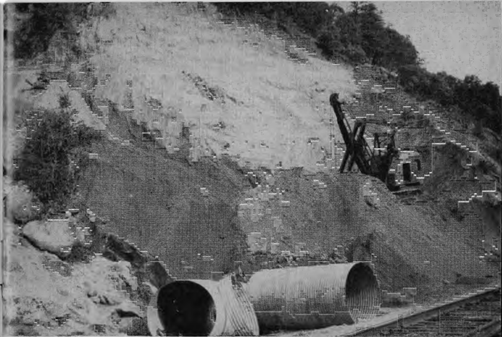
Right: Looking east, facing off for west portal of proposed Tunnel 15, January 12, 1956.
