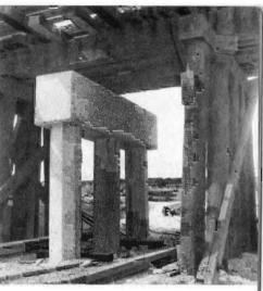
Above: prestressed piles and stringer in place prior to removal of old wooden structure.
