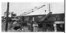
Above: Crane was used to remove old wooden structure, and (below) to drop new prestressed girder into place.
