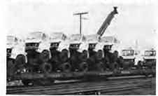
The crew just finished loading pedestal-mounted imported trucks for an experimental load to Maryland. The flat car came in with International Harvester trucks, and WP is using it with their permission in order to get a two-way haul. Photo by Norm Schlinger.
