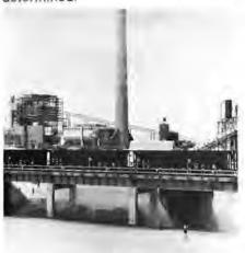
As the coal unit train moves across the trestle its cars are automatically unloaded through dump bottom doors. Nozzles under the trestle spray the coal with water to prevent dust. The train will make three deliveries a week at the North Valmy Generating Station in Nevada. (Union Pacific Railroad photo)
