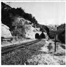
MILEPOST 250: A view of the east portal of Tunnel 15. Tunnel 15 is 3117.8 feet long and was constructed in 1956 after the massive flood of 1955.
