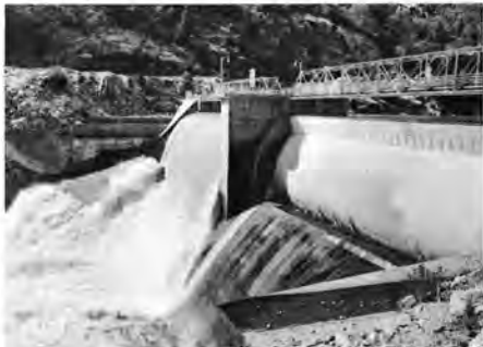
Cresta Dam, near WP mile-post #247, on the Feather River. The water captured behind Cresta Dam, which is 113 feet high and 384 feet long, flows through four miles of pressure tunnel which is 26 feet in diameter.
