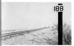
Milepost 188: Main line runs through here on an 18.14 mile straight line tangent,
