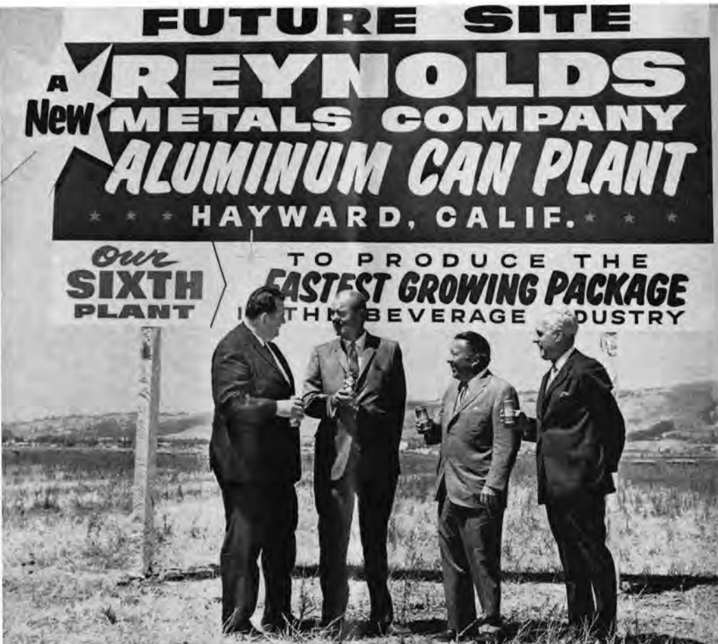
To toast the success of Reynolds Metals Co. sixth aluminum can plant, a 200,000-square-foot structure to be completed late next year, this group of executives scooped up dirt from the 20-acre site in Hayward during July. Left to right they are Mayor John K. Smith of Hay-
