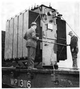
At Milpitas Cliff and Lead Carman Ed Churchill measured Federal Pacific Electric Co. transformers for high-wide load clearances.
