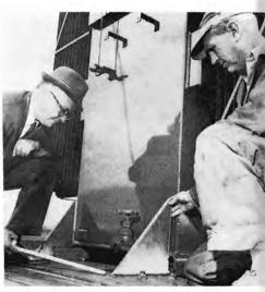
They then checked and found that gusset plates were uniformly placed to best support and anchor the transformer to car deck.
