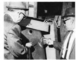
Another example of improper packaging that caused damage to this tub. This has since been corrected by having shipper use a wooden frame to better distribute forces encountered while shipments are in transit.
