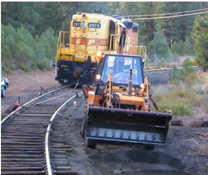
Some views from the Oct 24 - 25 track session. Our hardworking crews jack, align and reballast the balloon loop, aided by some of our locos and heavy machinery. -Wayne Monger photos
