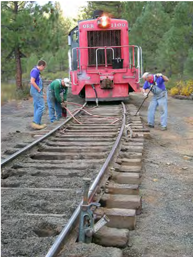
Some views from the Oct 24 - 25 track session. Our hardworking crews jack, align and reballast the balloon loop, aided by some of our locos and heavy machinery. -Wayne Monger photos
