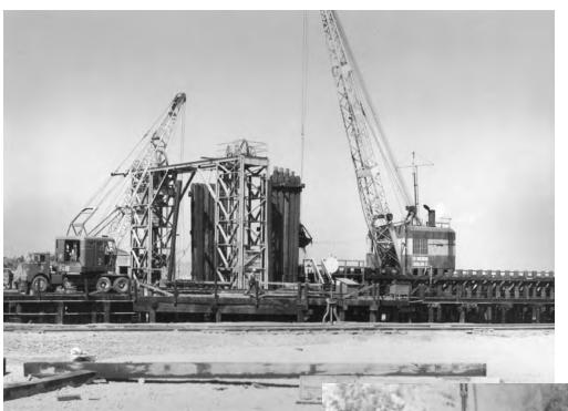
Here we have a rare shot of a ferry slip under construction. This is believed to be the Oakland slip, which soon sport a building for passenger transfer. That service would end in 1933 when the WP started running passenger trains into the SP Oakland Mole and the slip would be used solely for freight traffic until the end of ferry service on the Bay in the late 1970's.
