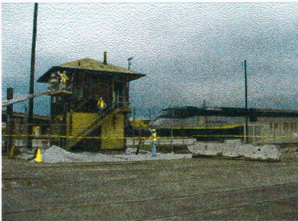
Photos of Magnolia Tower taken Wednesday, April 17.
