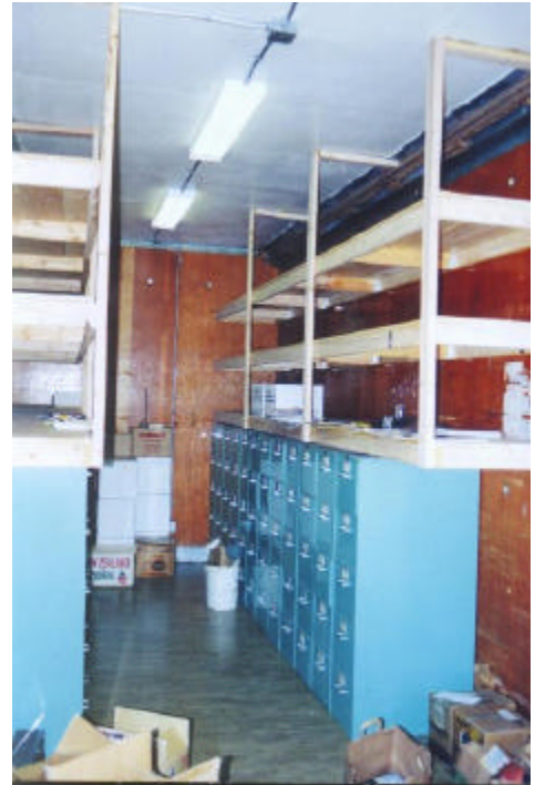
Overhead wooden racks provide box storage while books and magazines will be stored on metal shelving. Overhead and under rack lighting provide for a pleasant work environment.
