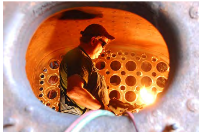
Steam CMO Chris Allan performs some welding work inside the 165's firebox.
