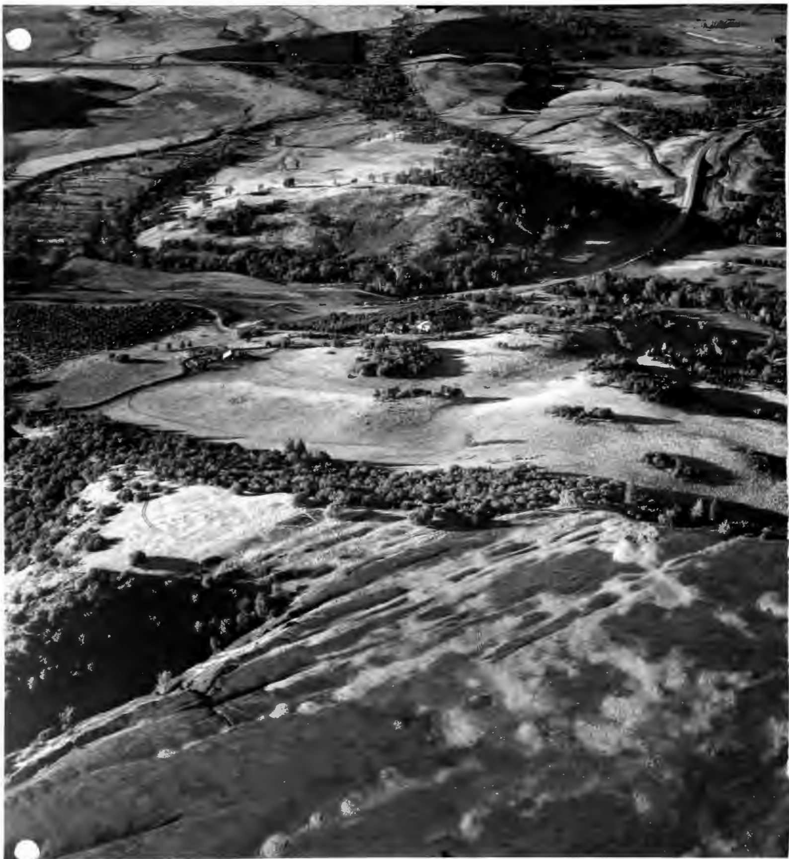
No. 1174-49 12-8-61 Oro Pentz Grading - Dodge Slide Area.
