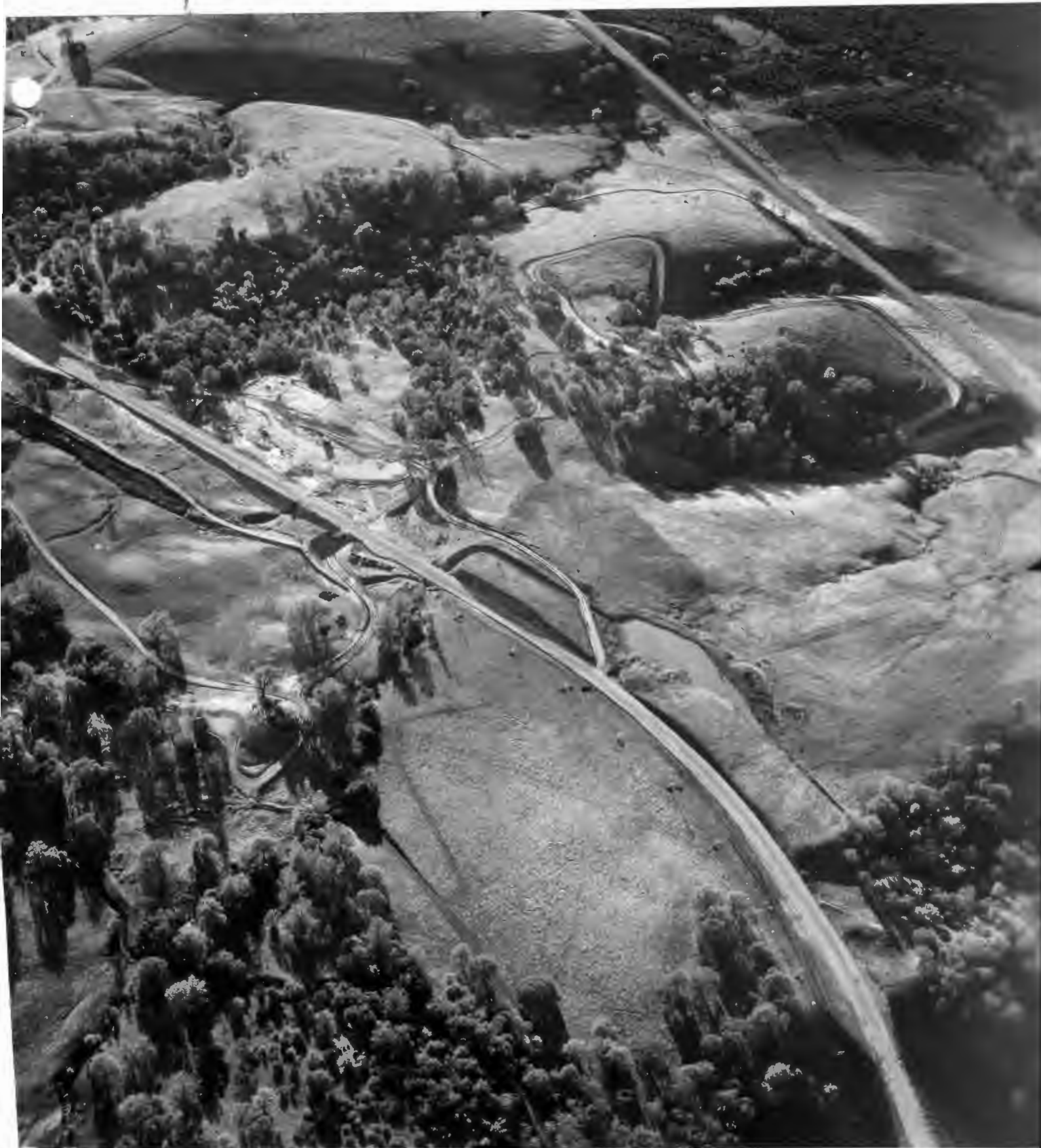
No. 1174-53 12-8-61 Oro Pentz Grading. Aerial view of Wheellock's reservoir and access road to Wheellock pit.
