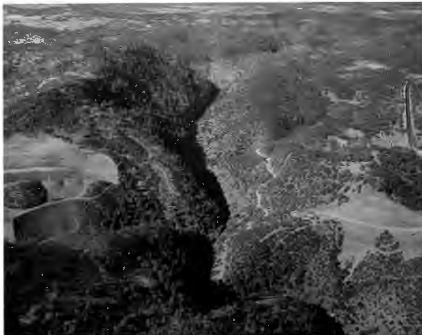
No. 542-1 11-25-59 West Branch Bridge. Aerial view of bridge site looking west.
