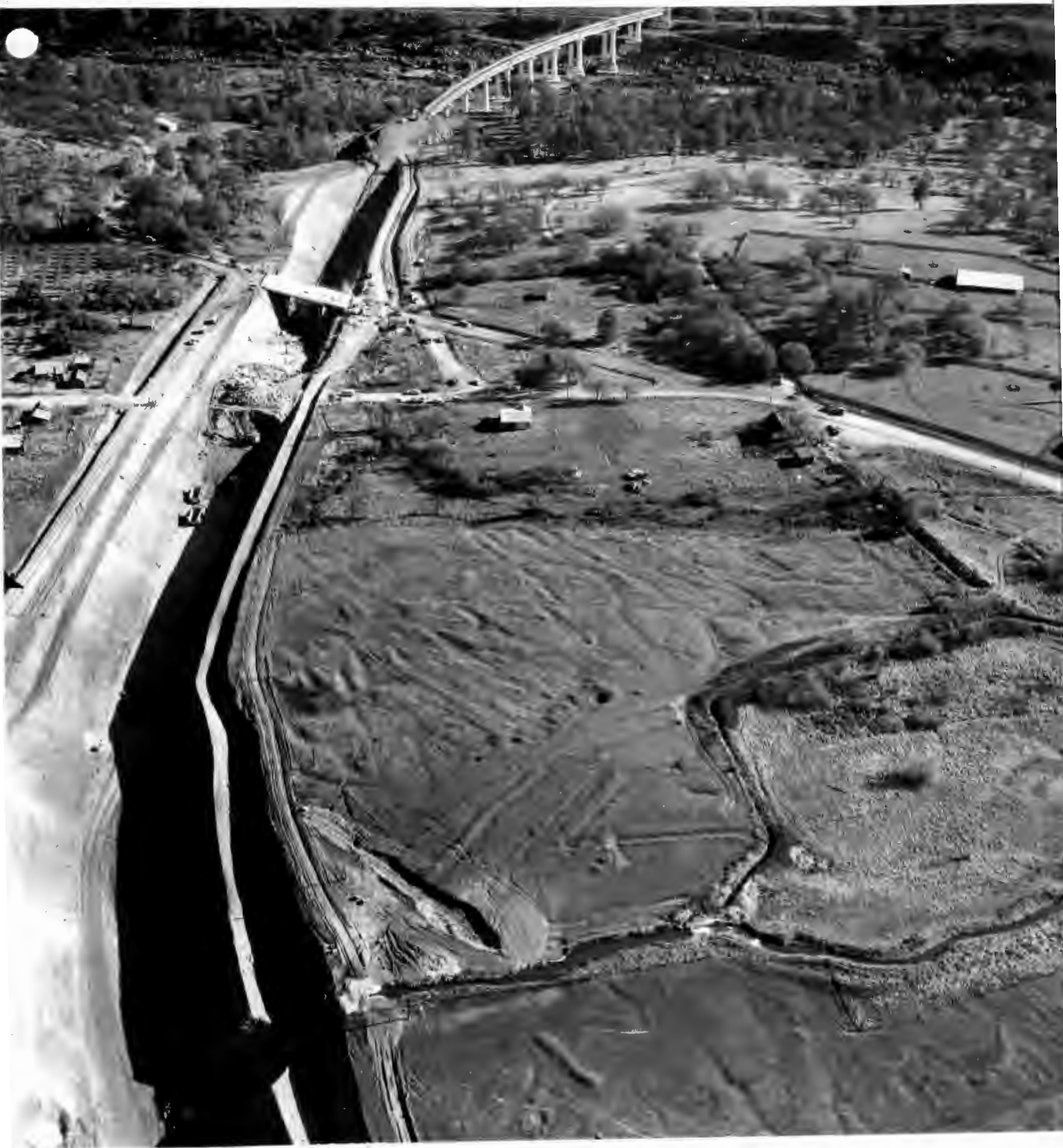
No. 1185-19 1-16-62 Oro Pentz Grading. Excavating cut in Thompson Flat.
