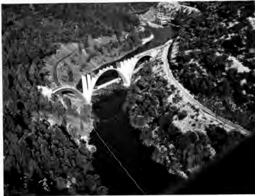
No. 560-5 1-15-60 North Fork Bridge. Aerial view of bridge showing access road on right bank of Feather River.
