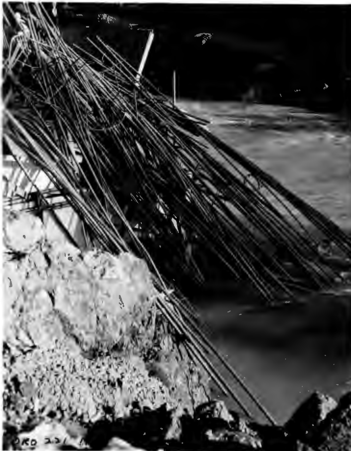
No. 221 1-13-59 Feather River Bridge Pier No. 4. Close-up of No. 18 bar steel lying in river.
