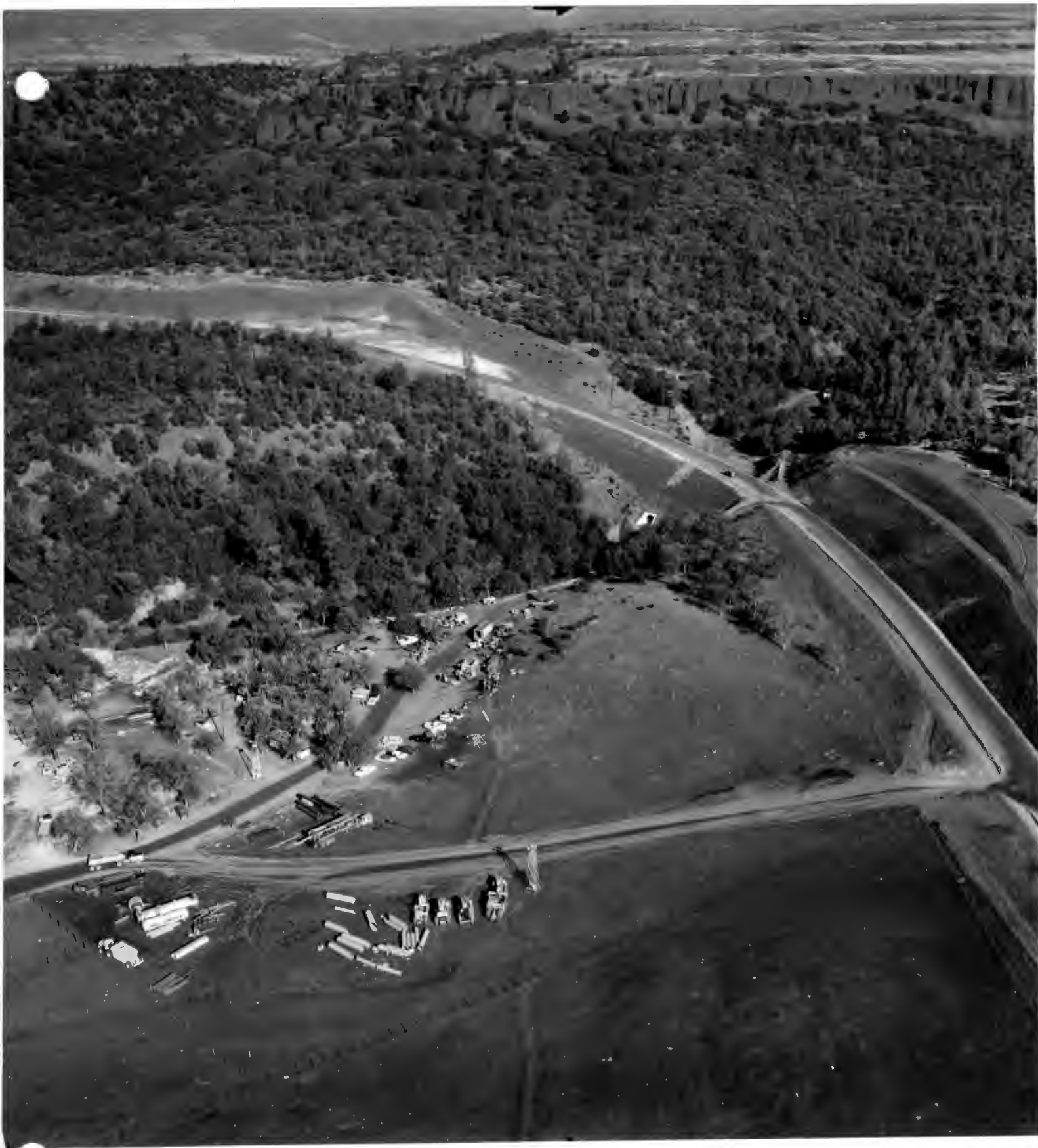
No. 1185-25 1-16-62 Oro Pentz Grading. Contractor's yard at Table Mountain Ranch.
