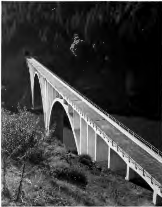
No. 859-2 12-5-60 North Fork Bridge looking toward Tunnel No. 5. East Portal Bridge is completed and ready for ballast and rails by Western Pacific.
