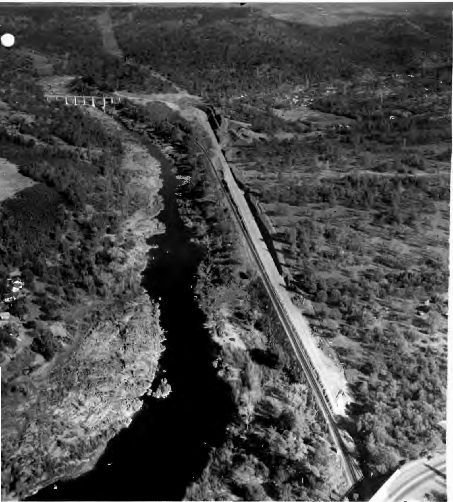
No. 1185-14 1-16-62 Oro Pentz Grading. Aerial view at east Oroville. Note subbase material in piles to be used when track is removed.
