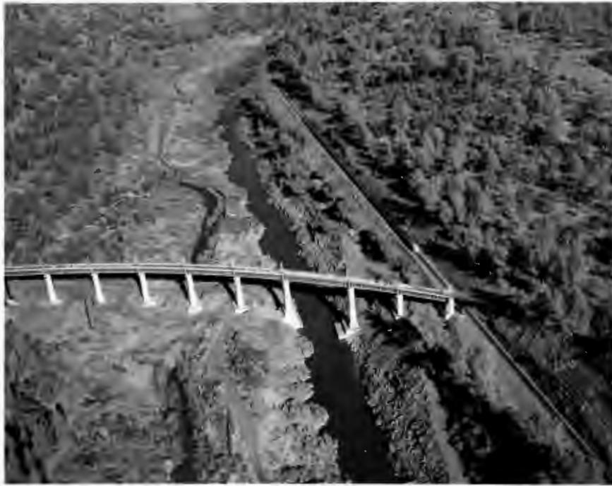
No. 559-1 1-15-60 Feather River Bridge looking upstream. Temporary crossing over existing W.P.R.R. tracks at far right.
