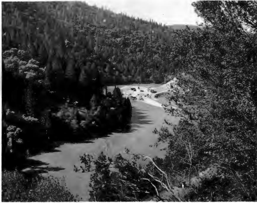
No. 118-5 4-22-58 North Fork Bridge looking upstream. Beginning at north side of low level crossing PG&E sandbar in center to be used as Contractor's yard.
