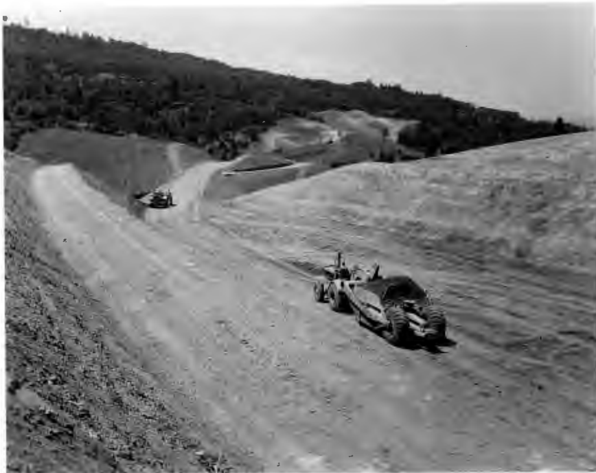
No. 1000-2 5-19-62. Oro Pentz Grading Job.
