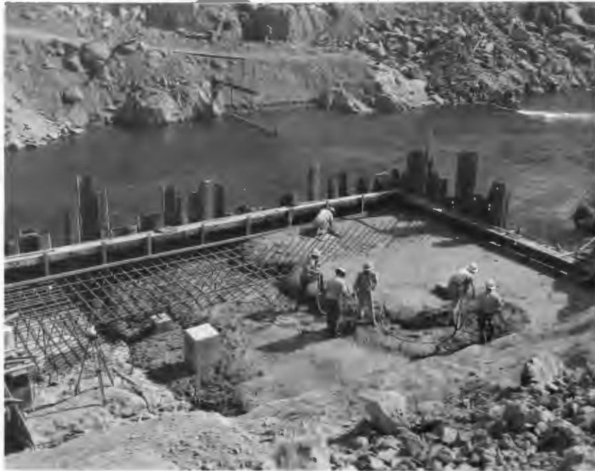
No. 189-3 10-16-58 Feather River Bridge. View back on line at concrete placing operation at Pier No. 4.
