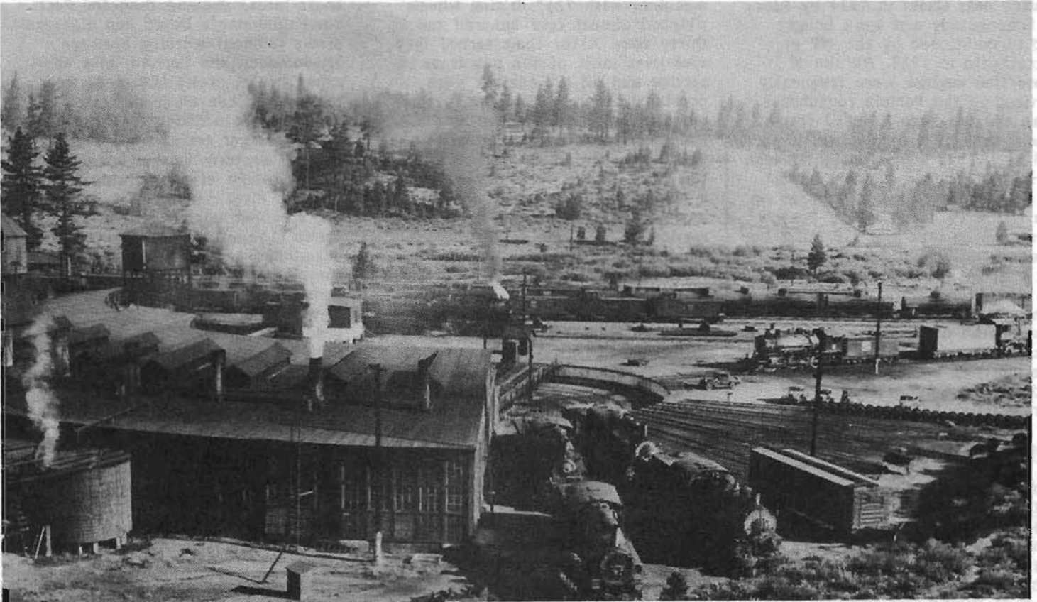
WESTERN PACIFIC RR ROUNDHOUSE AT PORTOLA IN 1939, LOOKING NORTHWARD
