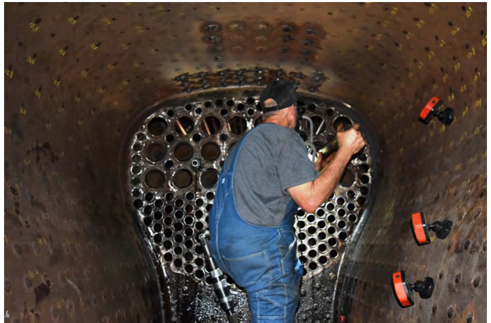
Roger is seen here in the firebox of the 165 with the super heater flues. All the flues are now in and cut the proper length. Next is to roll the ends and seal them.
