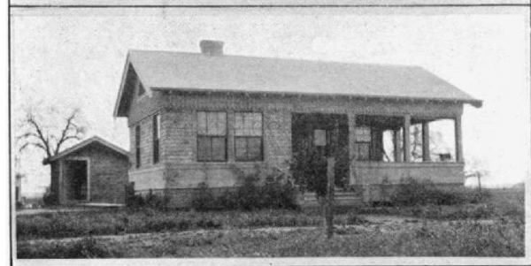
1. North Side of Nicolous Sub-Station. 2. Type of Cottage for Sub-Station Operators.
