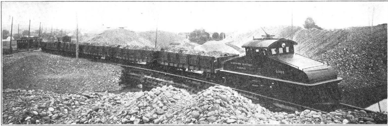
Hauling Rock for Ballast from Dredger Pits at Oroville.
